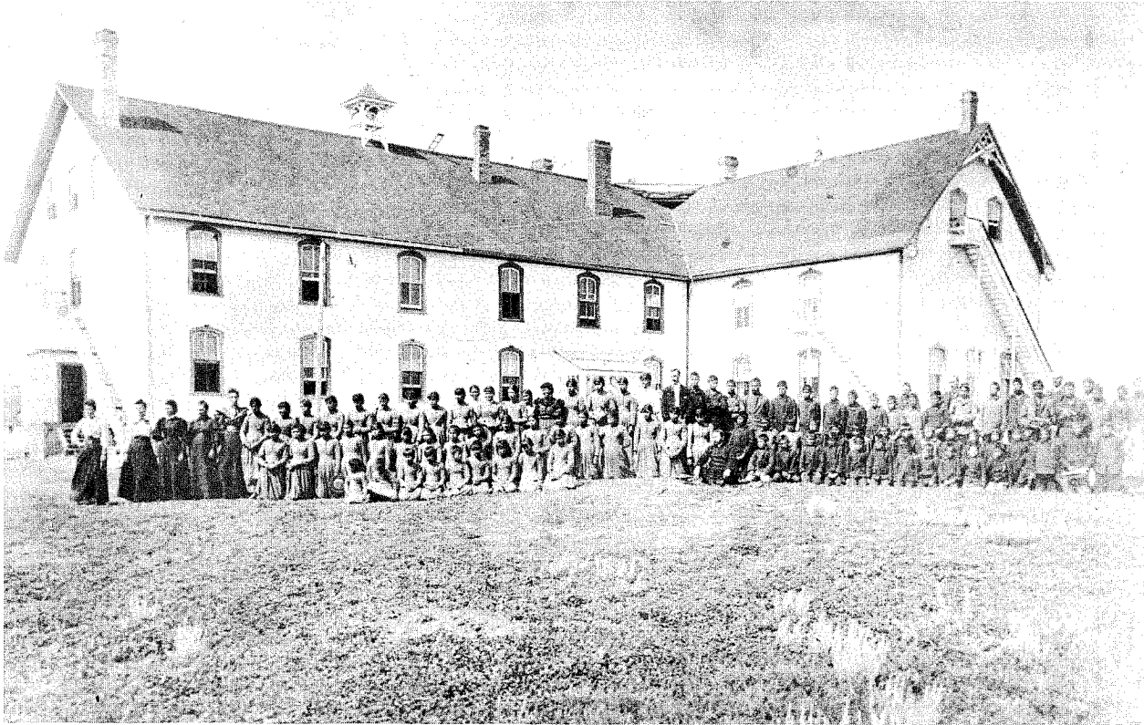
Note the number of chimneys, school bell, fire escapes. The roof is under repair.
