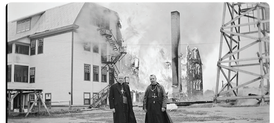
Sparks from a torch being used by maintenance staff during a repair job ignited a fire in the engine room of the Sturgeon Landing school. The fire quickly spread and burned the school to the ground. Photo: Mgr. Martin Lajeunesse O.M.I., R.P. Antonio Giard O.M.I. in front of the burning Sturgeon Landing School, on September 4, 1952, St. Boniface Historical Society Archives, The Roman Catholic Archdiocese of Keewatin—Le Pas/N3637
