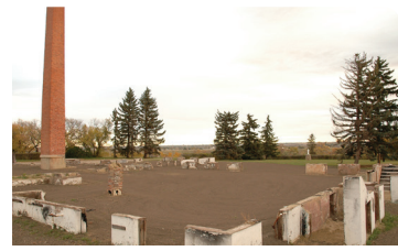
Stabilized ruins of the 2003 fire. Government of Saskatchewan, Photo by Calvin Fehr, 2004
