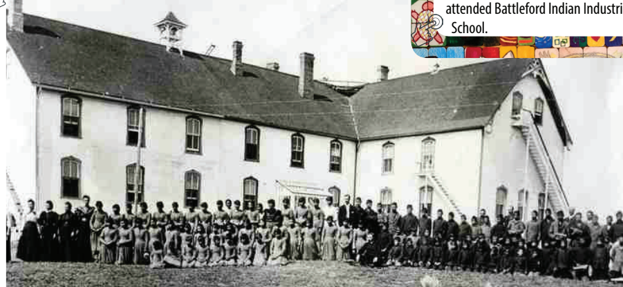
A photograph of the students and staff of the Battleford Industrial School taken by D. Cadzow, undated. Saskatchewan Archives Board Photo Collection/S-B 70
