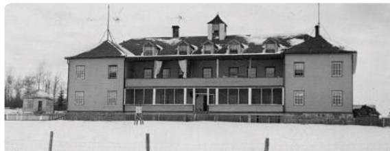
All Saints, Lac La Ronge (1907 - 1947) destroyed by fire (The General Synod, Anglican Church of Canada, MSCC/P7538)
